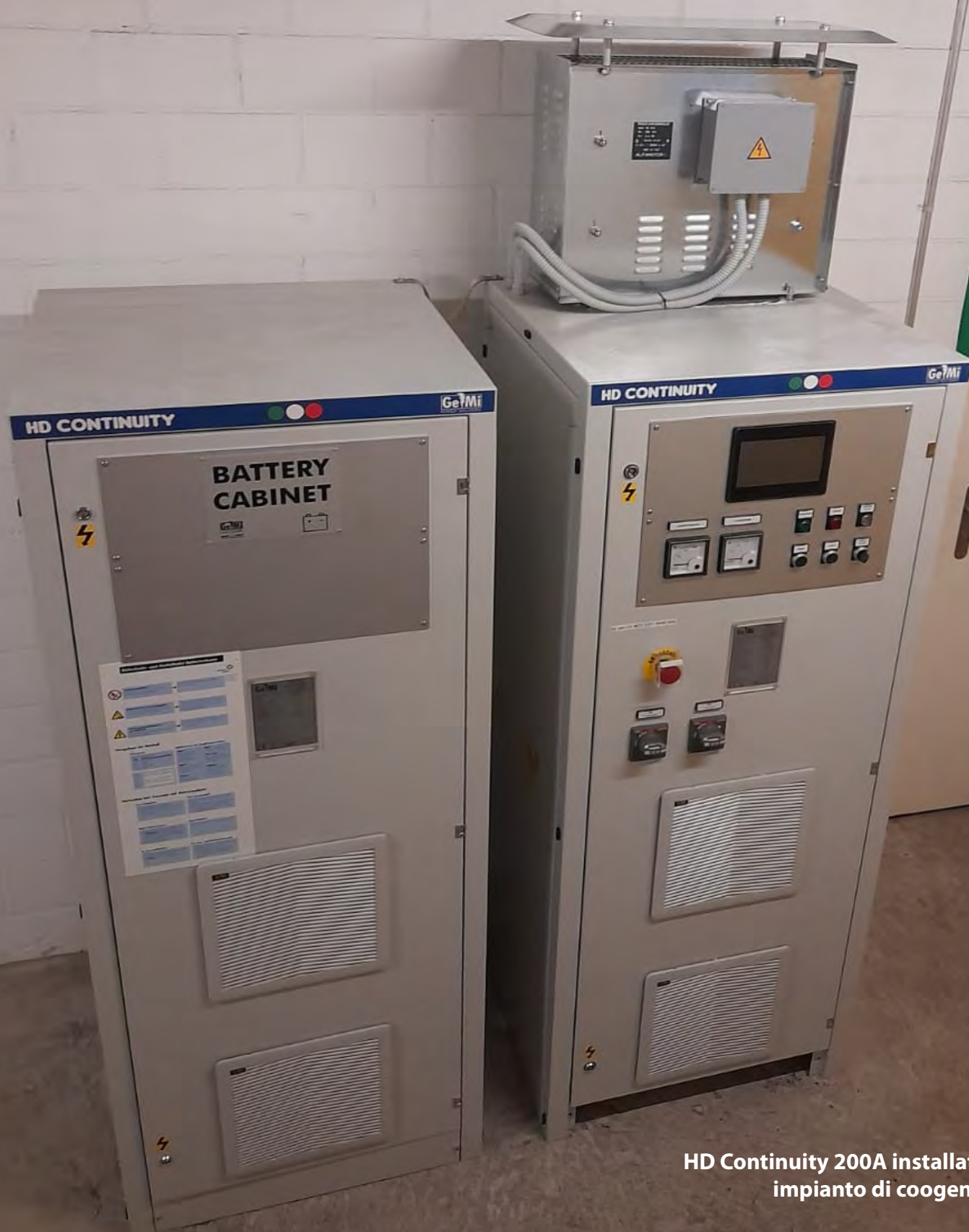
HD Continuity 200A installed in co generation plant
